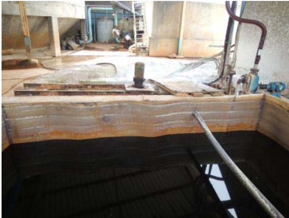
Figure 3. pH regulation system on a textile mil ETP (Zhejiang Lifeng. 100 m 3 /h)
