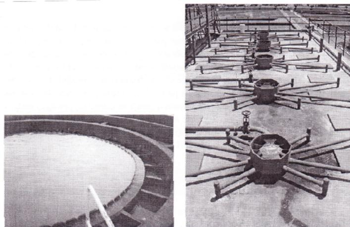
**Figure 3.- Influent distribution structures in: (a) a circular reactor (left side) and (b) a rectangular reactor (right side).**
