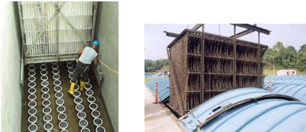
Figure 3.- Rope fixed support Ringlace. Clean (left); colonized by biofilm (right)
