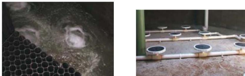
**Figure 6.- Left: BIO-BLOK filling media assembly, where coarse bubble aeration is observed. Right: diffuser assembly.**
