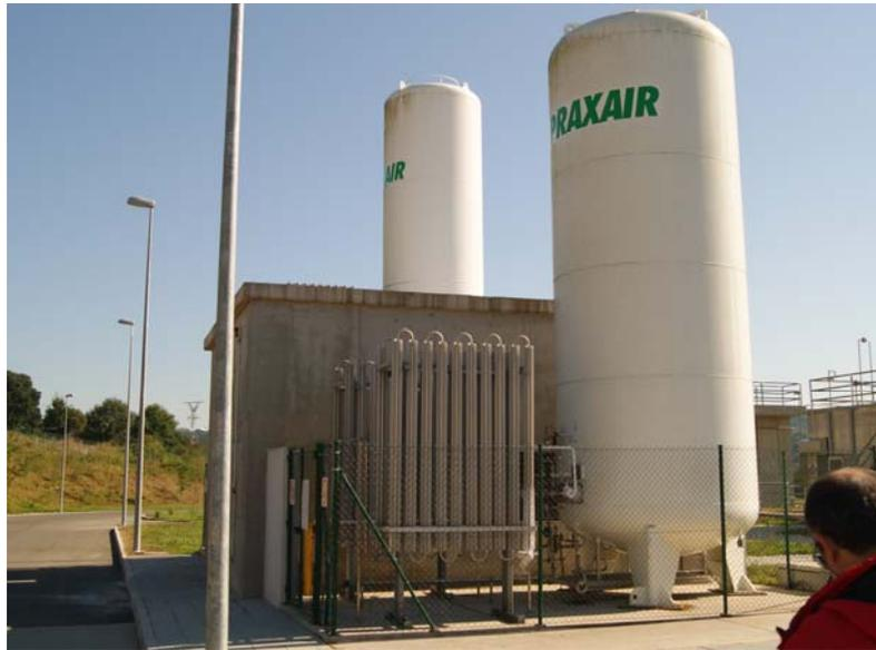
Figure 1.- Cooling system and oxygen storage (ETAP-Lugo).
