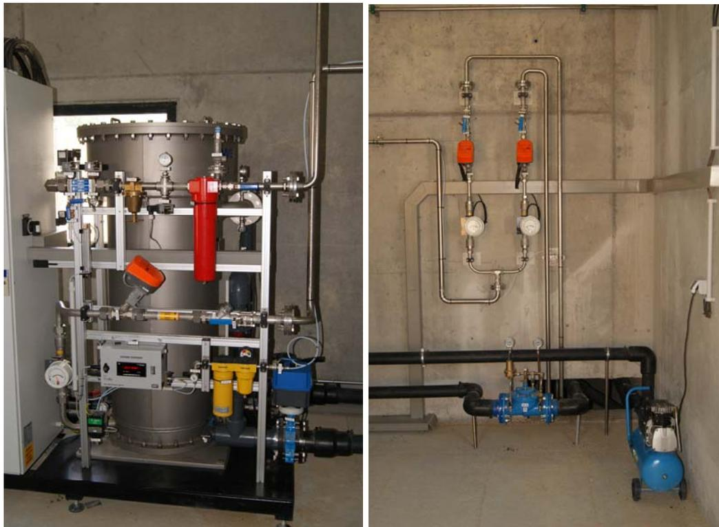
Figure 2.- In-situ ozone generation equipment (left) and pressure and gas controllers (right). ETAP-Lugo.
