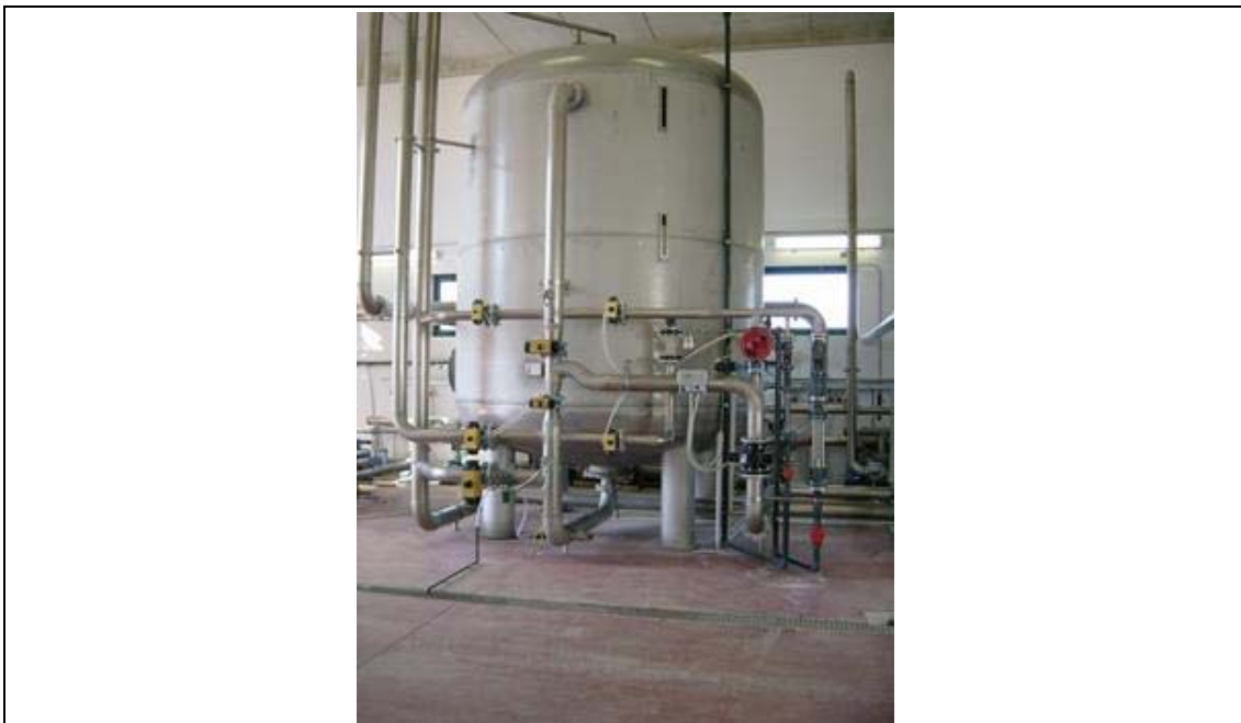
Figure 2.- Single column ion exchange unit (Europrogetti Recovery Water Technology www.europrogetti-italy.com )
