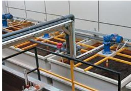
**Figure 2. Industrial wastewater treatment using advanced oxidation Fenton process. Reagents required in each stage are supplied to successive reactors from storage tanks in a fully automated treatment process. The compactness of the system is enhanced by the use of lamellar sedimentation units. (Source: TECNA, s.l.r., Italy, [www.tecna-italy.com](http://www.tecna-italy.com))**
