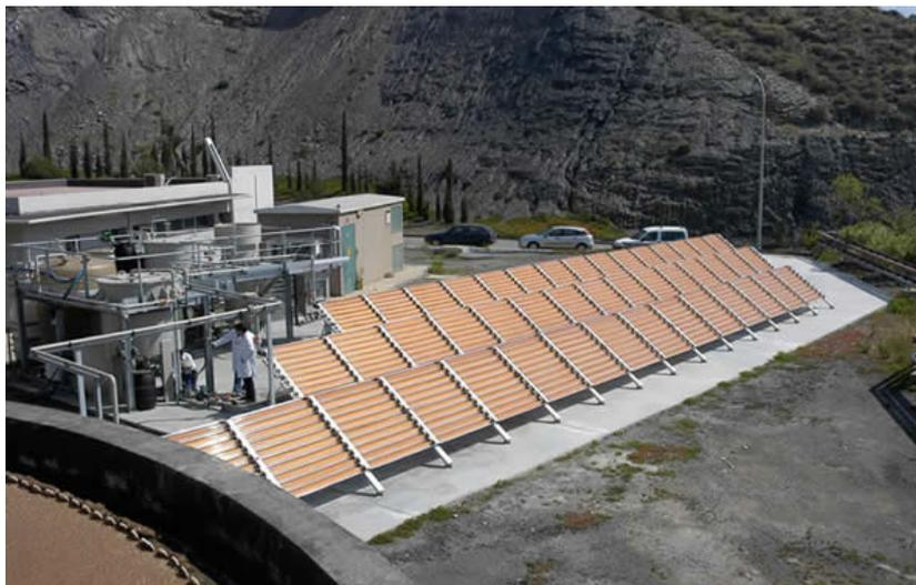
**Figure 7. Solar Photo-Fenton facilities in Albaida, S. L. in La Mojonera (Almería, Spain), dedicated to pesticide waste washing water treatment. Please observe the reddish tone caused by Fe (III) precipitates ([www.psa.es](http://www.psa.es)).**
