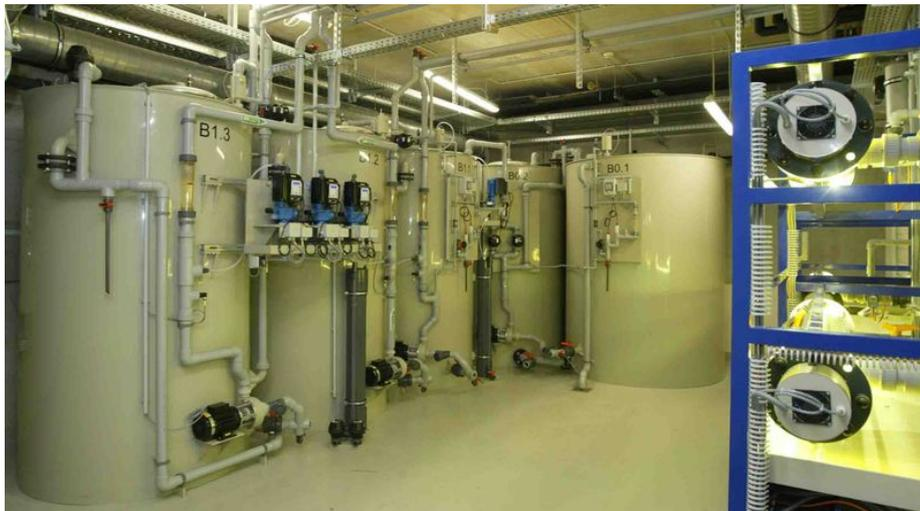
**Figure 6. UV Photo-Fenton treatment system applied to an industrial effluent tertiary treatment (Ref.: Enviolet GmbH, Karlsruhe).**
