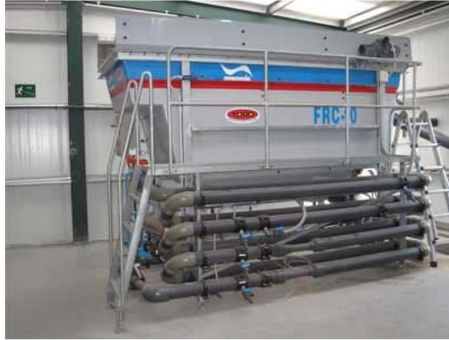
Figure 14.- DAF system with prior flocculator tube (Float Anaconda® FRC-20; 20 m<sup>3</sup> / h; TORO).
