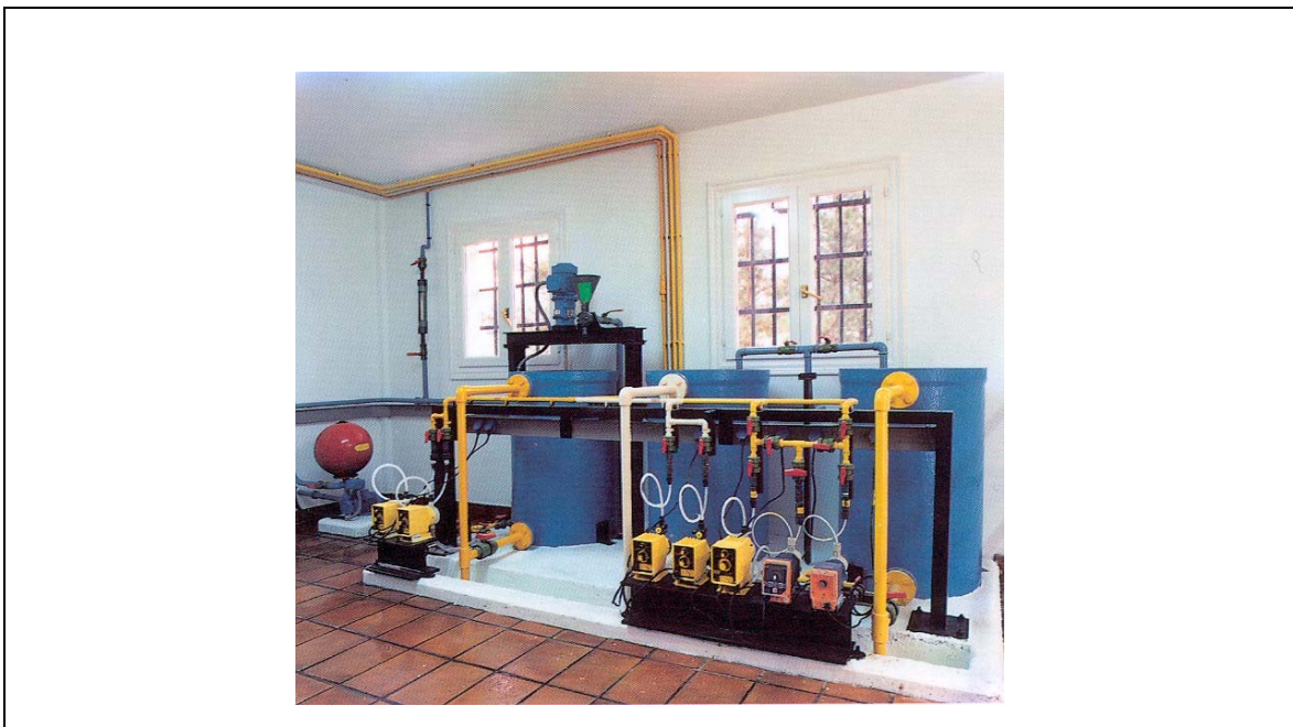
Figure 12 Reagents preparation and dosing system.
