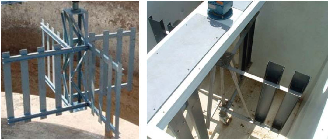
Figure 7 Flocculation stirring paddles.
