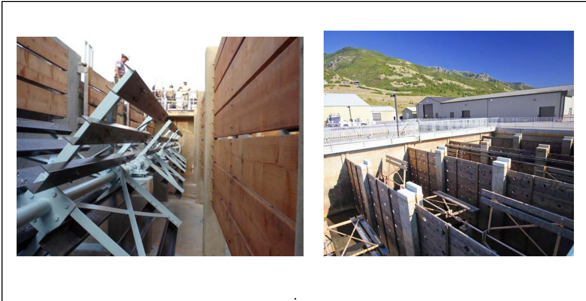
Figure 9 Plates for slow agitation in flocculation chamber with horizontal axis. (WesTech).
