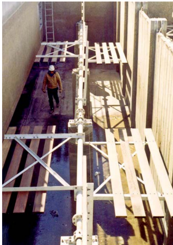
Figure 8 Paddles for slow agitation in a flocculation chamber with horizontal axis. (WesTech)..
