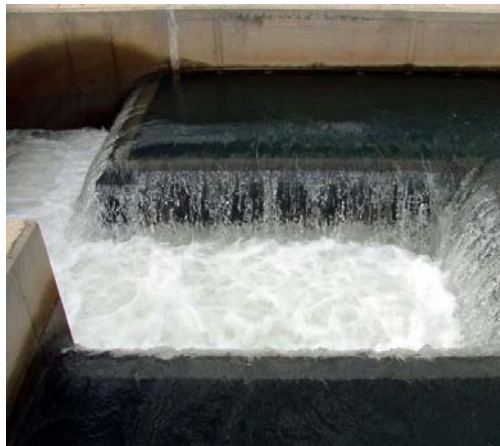
Figure 5 Mixing system and coagulation by hydraulic jump.
