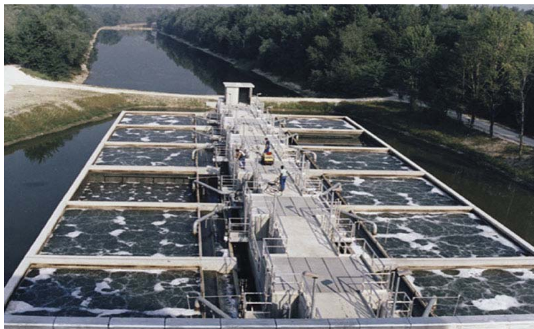
Figure 2.- Aerated biofilter system of technology Biofor
