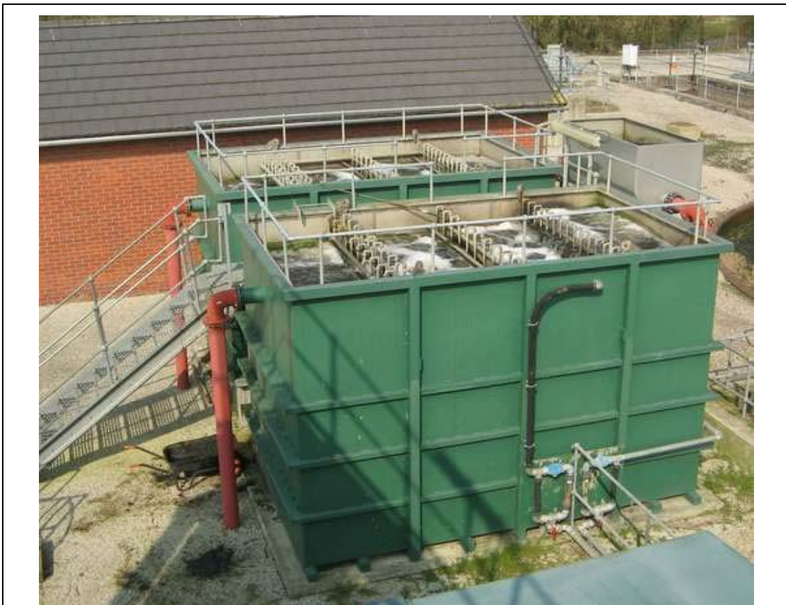
Figure 4.- Aerated biofilter system prefabricated metal structure for flow rates up to 1000 \text{ m}^3/\text{d} .
