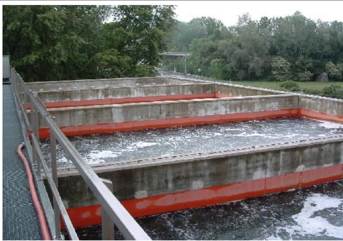
Figure 1.- The biofilter system technology Biostyr
