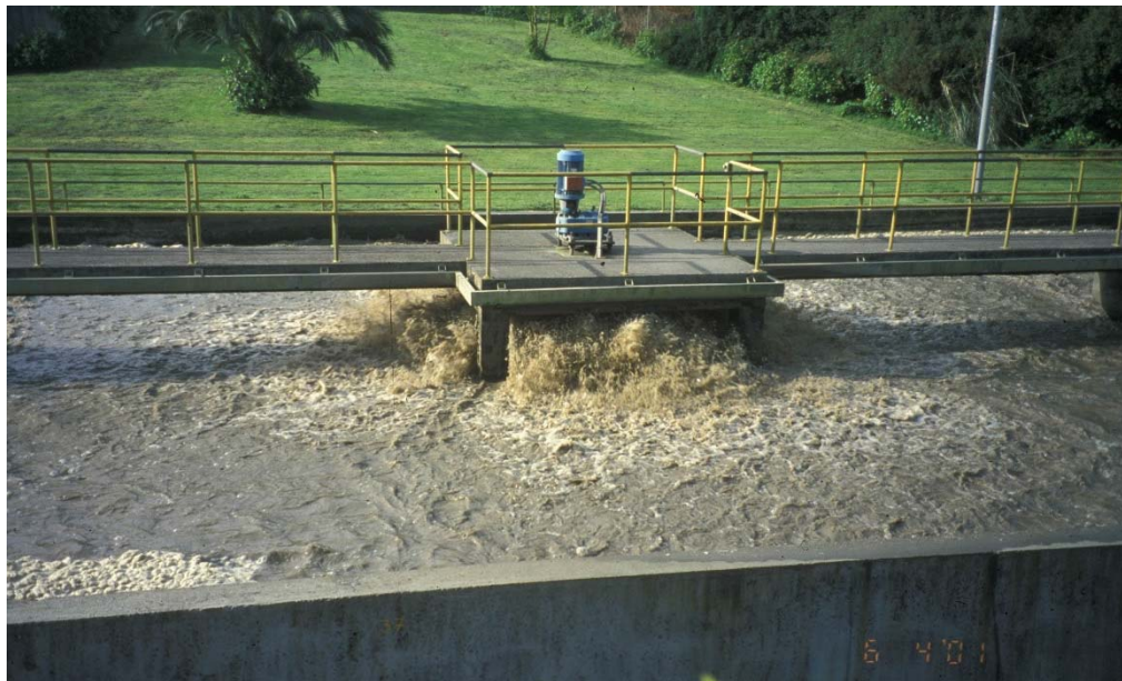
Figure 2 Activated sludge reactor. Industrial ETP at Bergondo (Spain).
